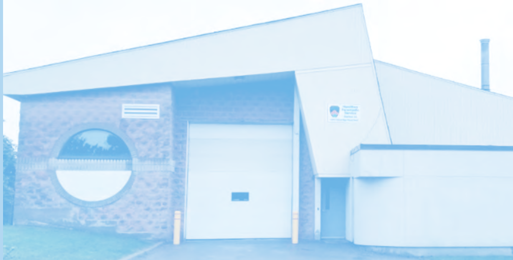
HPS Station 32, Limeridge Rd. E, Hamilton
